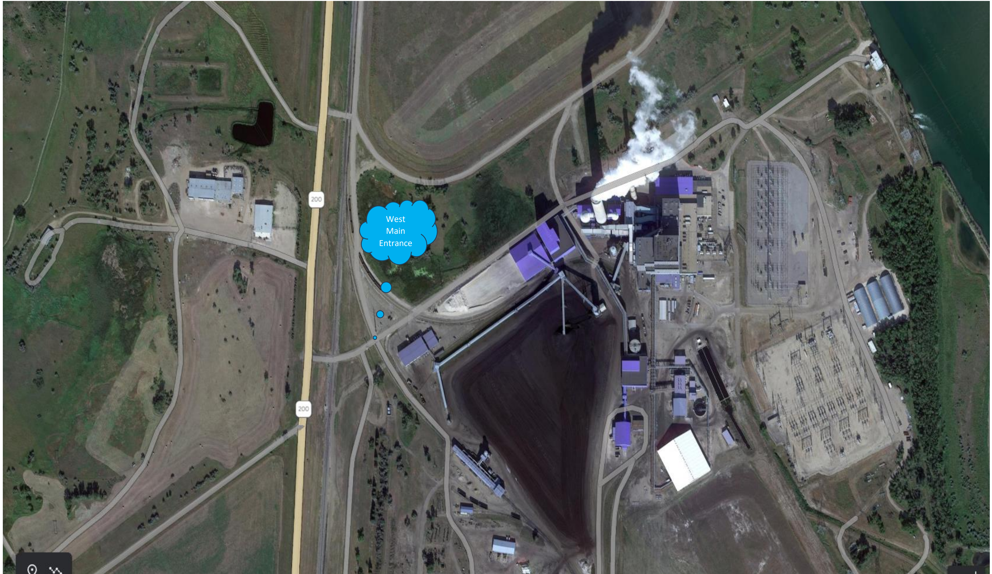
Leland Olds Station: Aerial view 8-17-23
